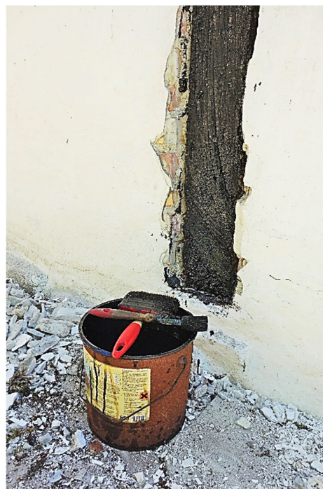
The light brown wood tar is slightly heated and brushed onto the soft areas of the timber with a brush. You can subsequently brush over all the timber, if this has been completely cleaned of paint, lime etc. You can also advantageously mix pigments in the hot wood tar, so that the wood becomes harder after hardening.
