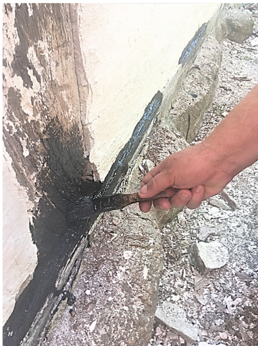
The light brown wood tar is slightly heated and brushed onto the soft areas of the timber with a brush. You can subsequently brush over all the timber, if this has been completely cleaned of paint, lime etc. You can also advantageously mix pigments in the hot wood tar, so that the wood becomes harder after hardening.
