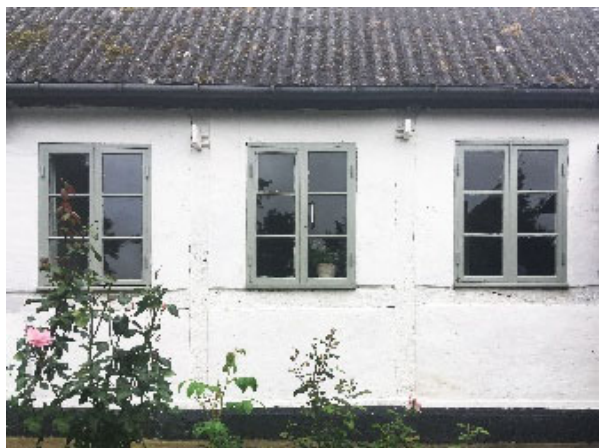
Photo series of half-timbered facade restored through biochemical consolidation of the wood with wood tar color. Møllestangsvej 9 at Nyord in Denmark.
