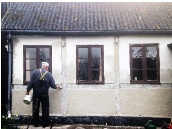
Photo series of half-timbered facade restored through biochemical consolidation of the wood with wood tar color. Møllestangsvej 9 at Nyord in Denmark.
