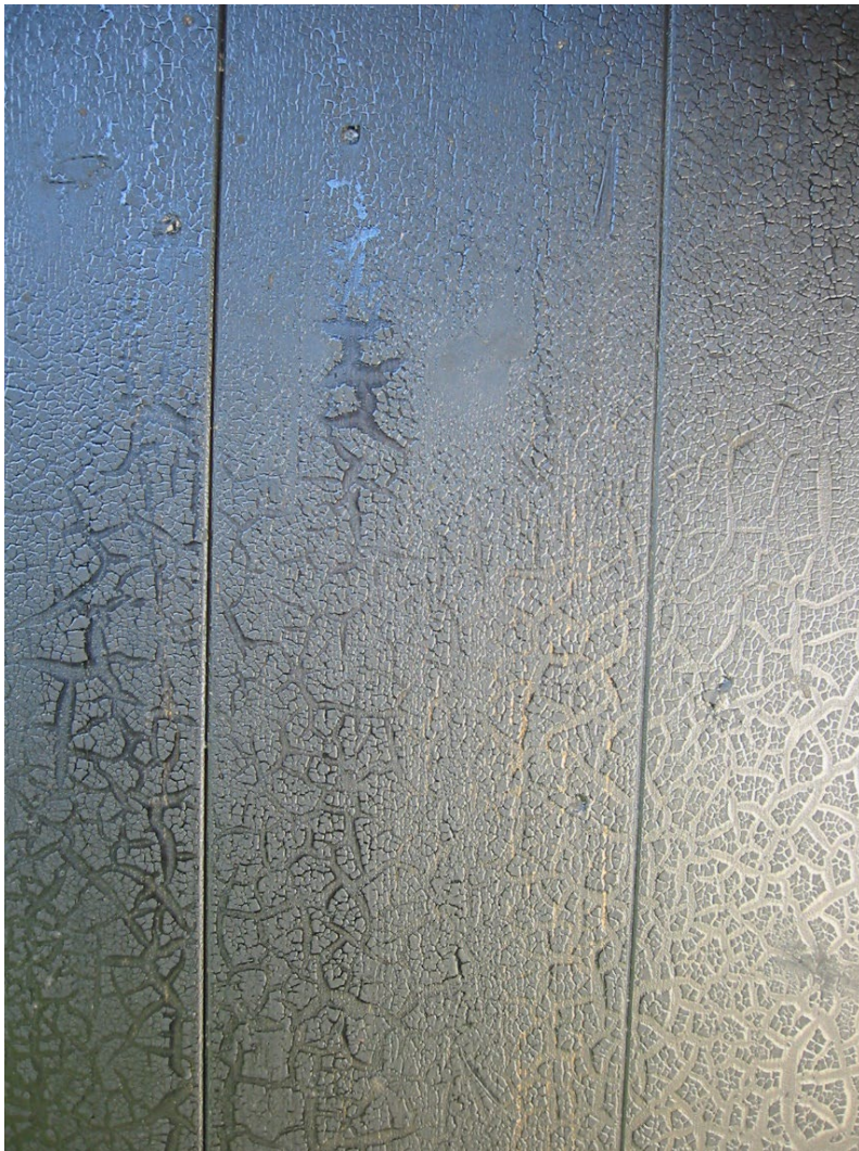
The wood tar colour, here with black pigment, makes after some time very characteristic patterns, called 'elephant skin'
