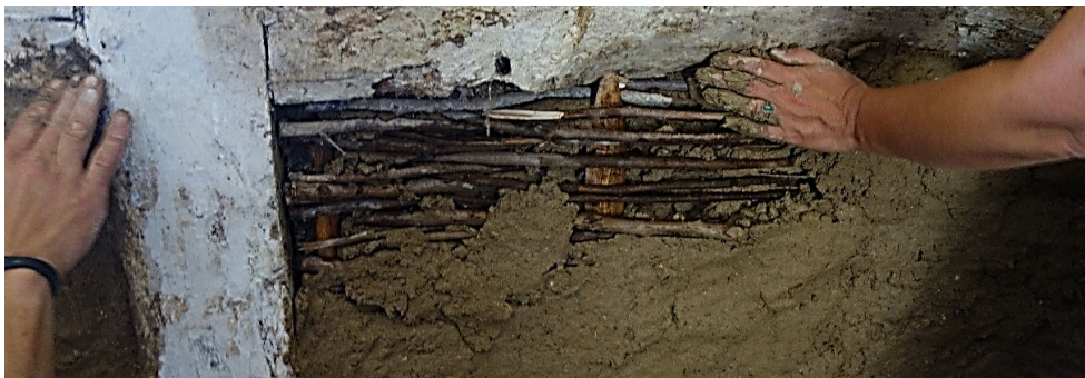
Clay cladding of half-timbering on hazel cane
