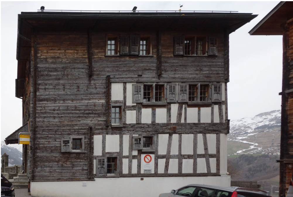
FIG 3: Building in Switzerland comprising both log construction and timber frame, both constructions are obvious of wood. (Photo: Søren Vadstrup)
